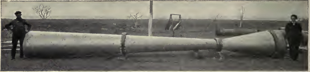
METER TUBE BEFORE INSTALLATION AT PUMPING STATION
